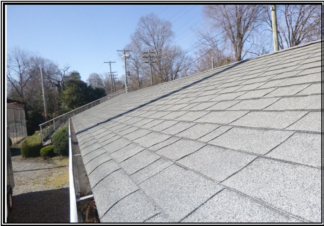
3. Suspect ACM – roofing materials – no asbestos identified
