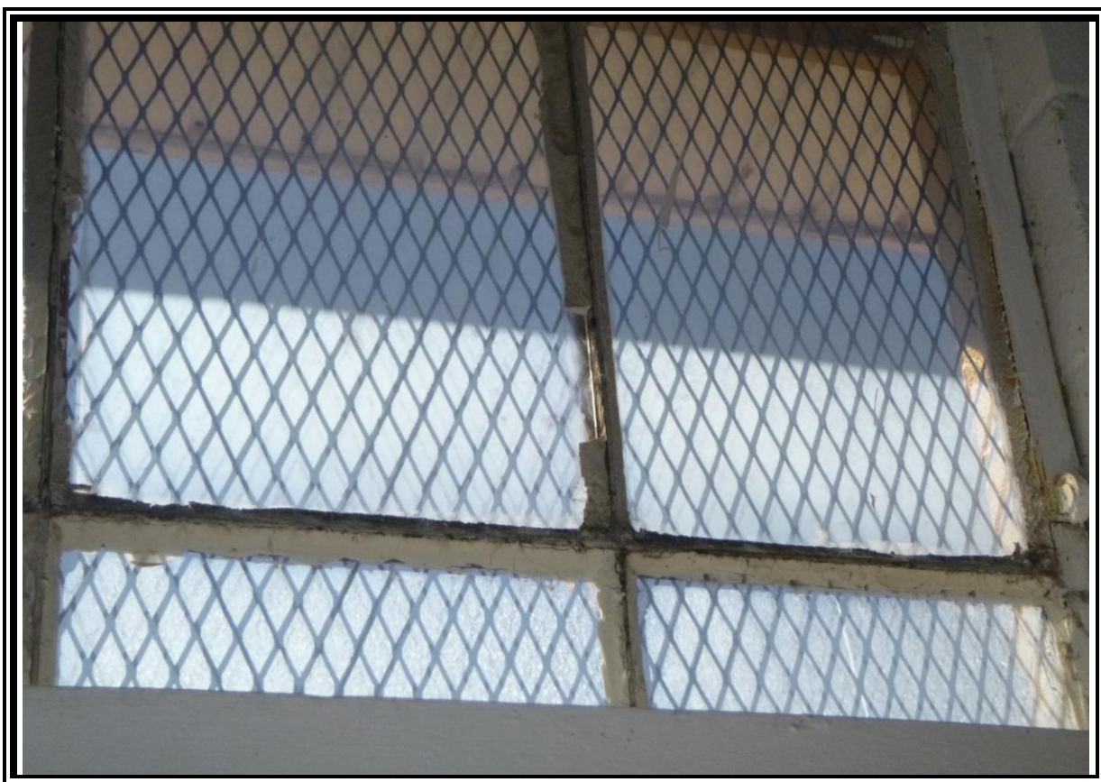
10. Suspect ACM – window glazing – no asbestos identified
