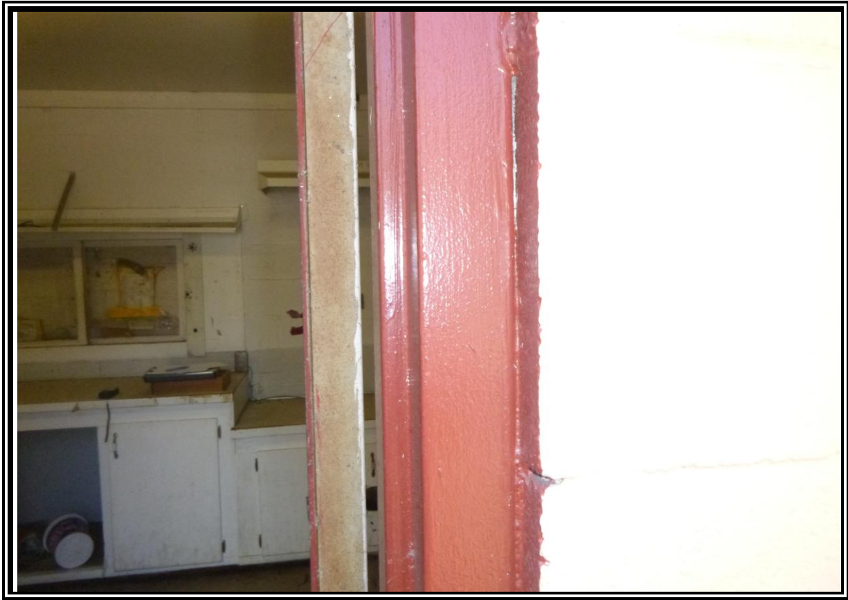
5. Suspect ACM – exterior door caulk – no asbestos identified
