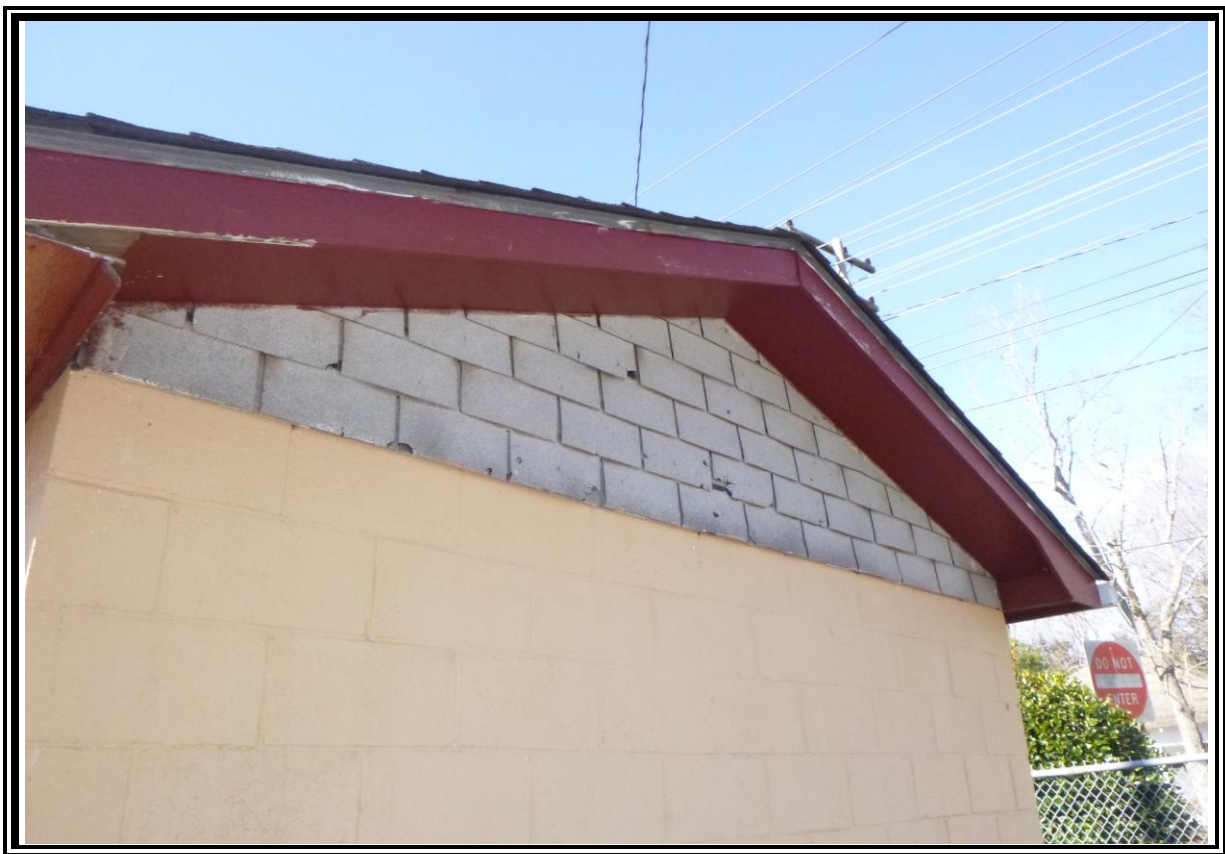
4. Suspect ACM – gable shingles – no asbestos identified
