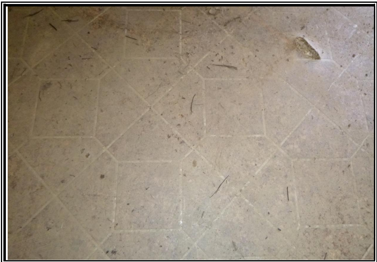
6. Suspect ACM – flooring materials – no asbestos identified
